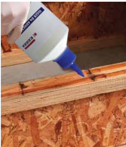
EGGER D4 Adhesive being applied following the Rapid Deck Floor Laying System
