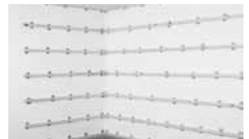
Wooden slates directly on the wall
