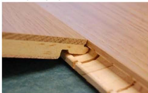
Installation of sports hall floor over battens supported by cradle supports Photo: Junckers
