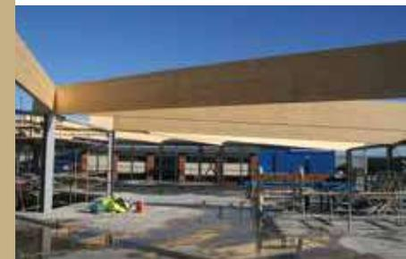
Glulam beams are a lightweight, eco-friendly alternative to concrete and steel beams providing an attractive natural look for large open spaces. Our large range of Glulam sizes can be used for a wide variety of applications including straight, angled and curved frameworks.
