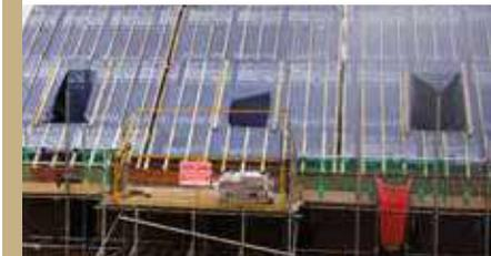
The fully designed and engineered panelised roof system offers an innovative and unique warm roof solution.
