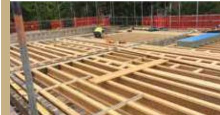
Our Steico I-Joists are designed in-house to individual requirements from one-off projects or roofs to full site plans and complex commercial structures.
