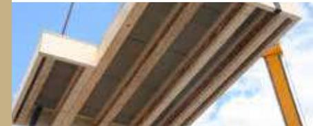
We manufacture both roof and floor cassettes which are ideal for faster build timber frame, which not only offer significant increases to the speed of build on site, they also significantly reduce time spent working at height.
