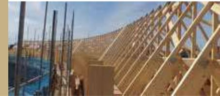
Supplied as fire and sound rated timber frame panels, made to the profile of the roof. Manufactured from a range of materials including plywood, OSB and plasterboard, the panels can be filled with solid-slab insulation and fire-treated as required.
