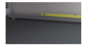
**5.** Fit additional feet at approximate spacings in between the first and last foot, and adjust for height.
